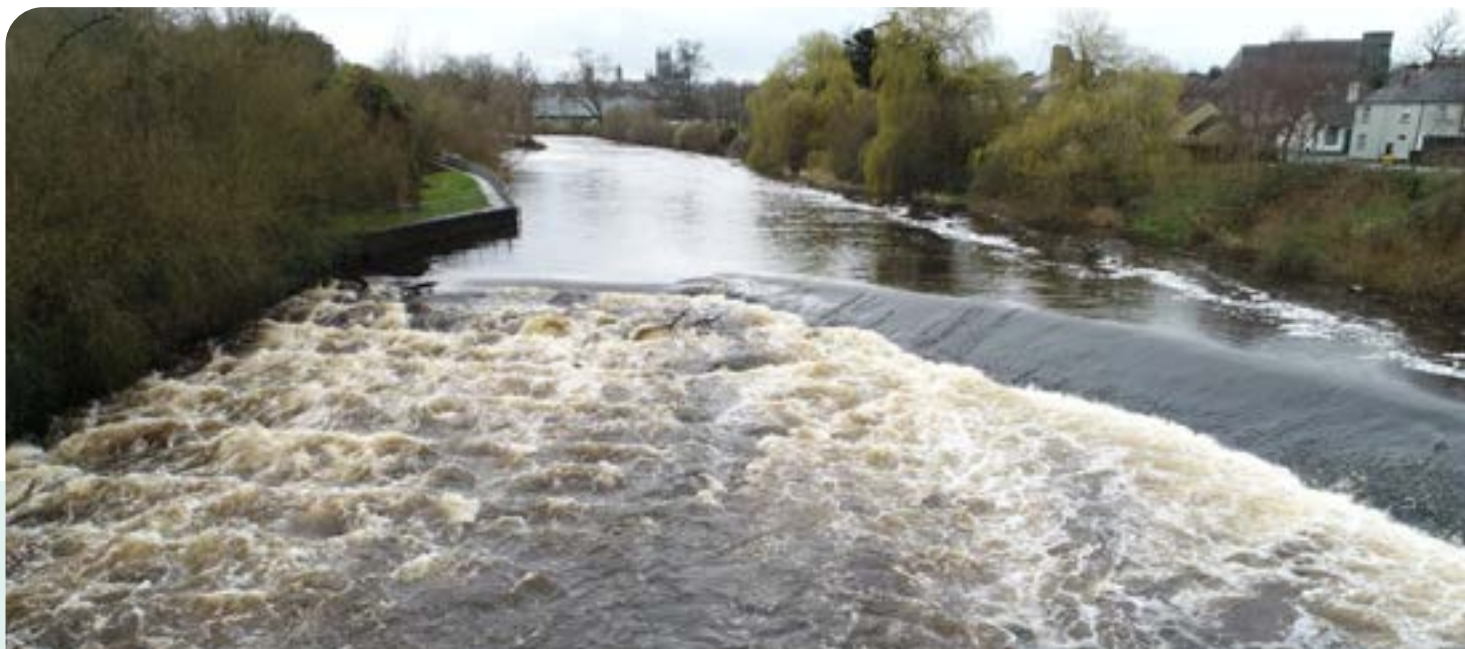
Fish pass placed to help Atlantic salmon and other fish species migrate over a weir on the River Nore – the footprint of the fish pass is visible to the left of the weir in picture as riffle water in a flood.
