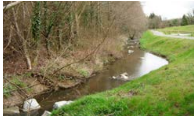
A pool with carefully placed boulders were placed to create hiding places for fish and areas where river birds such as wagtails can stand.
