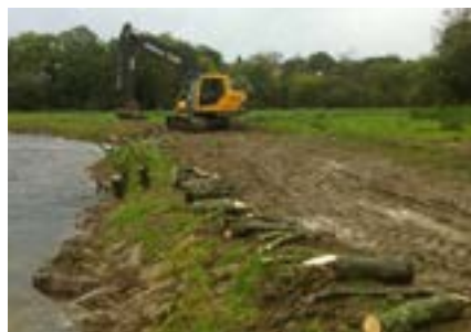
During works – working to reduce the rate of erosion by using a mixture of tree planting, rock and bank reprofiling. Large willow stakes are planted to bind the banks with their roots.
