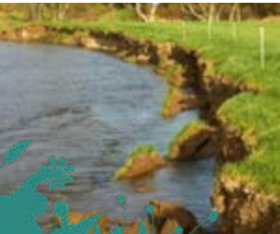
Before works - severely eroding river banks causing sedimentation of salmon and trout spawning habitat. A vulnerable population of threatened Freshwater Pearl Mussel is also being impacted downstream and the farmer is losing land.
