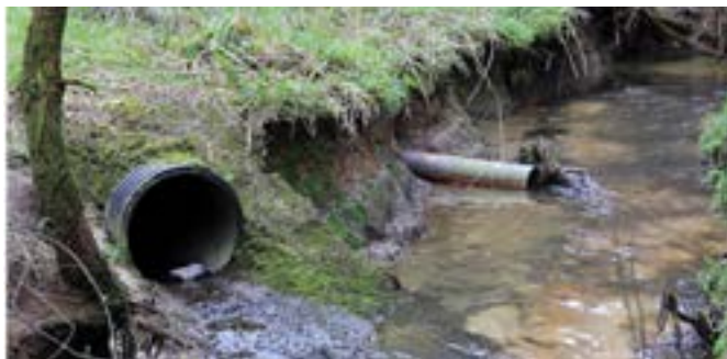
The impacted drain showing the absence of quality habitat for fish and other species.
