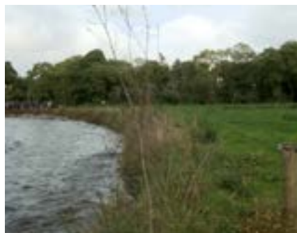
After works - two years after the work was completed, the river bank has completely naturalised. The willow trees and riparian vegetation have now grown up providing habitat for a range of wildlife and livestock are fenced off to prevent trampling of the banks and soiling of the water.
