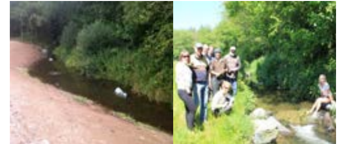
The river bank was reprofiled and a meander put in the stream. Rocks were introduced to increase the diversity of habitat in the stream and provide cover for fish.
