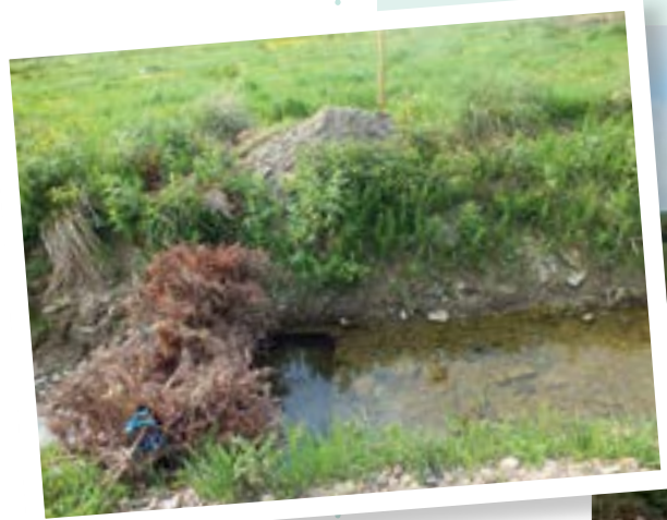
Silt trapping in a farm drain
